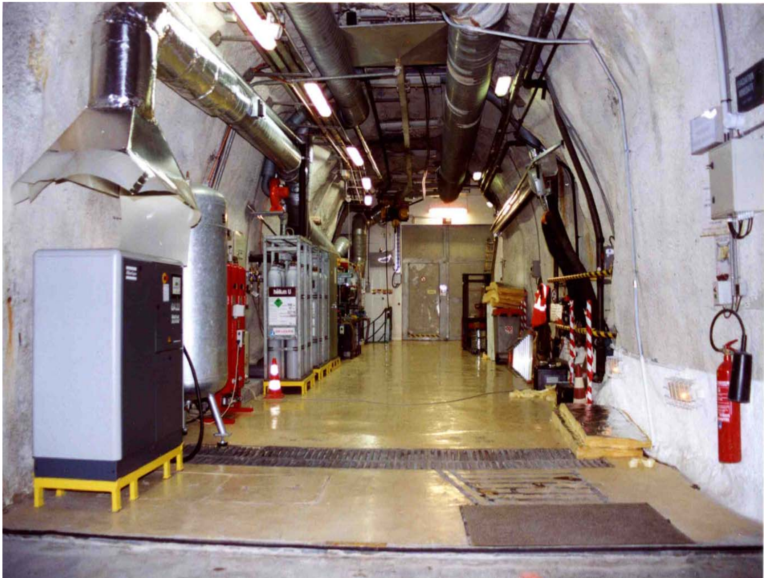
Air-lock between tunnel and lab
